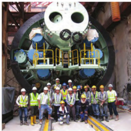
Contractor Yu Sin Engineering Work Pte Ltd sought a solution to move the boring machine parts over a distance of approximately 66ft (20m).
