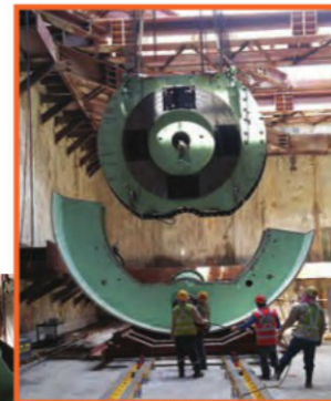
Another component arrives at the bottom of the shaft.
